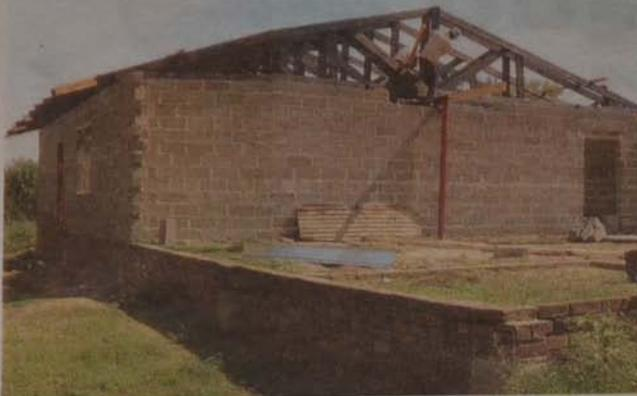
Day 21 - Finish mounting the timber that will hold the roof. The zinc, the ridging and the roof nails are delivered.
